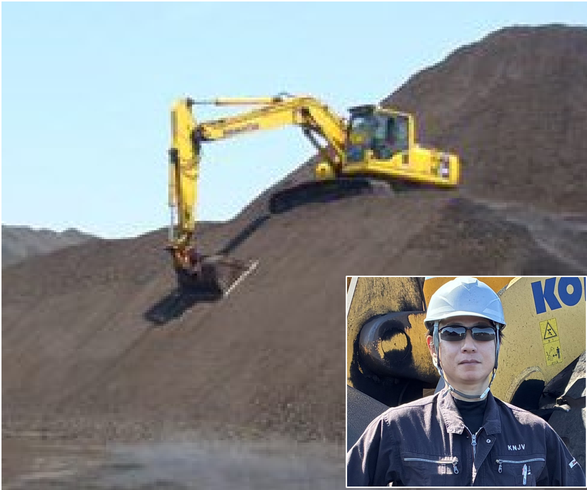
Compaction of stockpiles by skilled operators.
