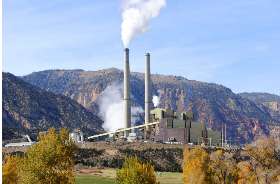
Huntington Power Plant
