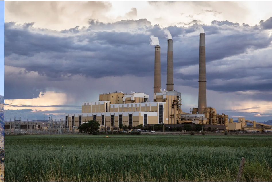
Hunter Power Plant
