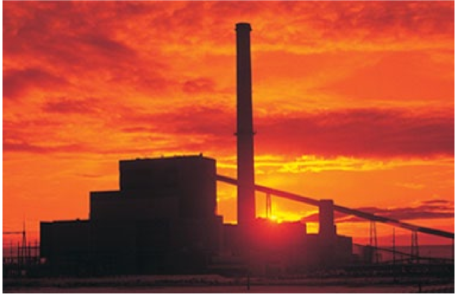
Bonanza Power Plant
