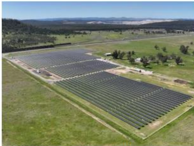
Solar power generation facility that has commenced operation
