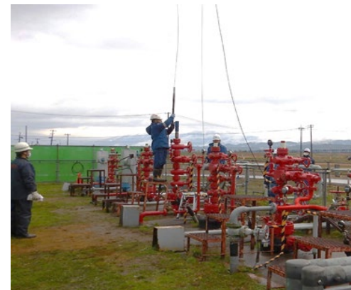
Fiber-optic Data Acquisition & Installation
