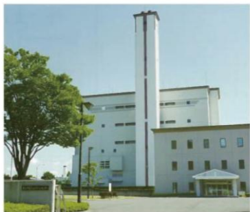
Fukuyama Waste Management Center (Koriyama city)
