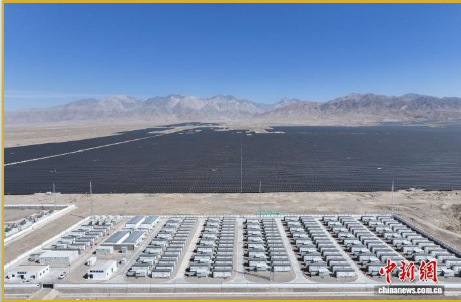
Qinghai Delingha PV-Hydrogen-Storage Integrated Project
